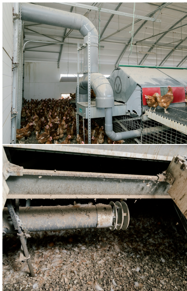
Image 9: Illustration of an ammonia scrubbing system in a poultry house, showing ducting, and air inlet immediately above the manure (Housing Measure 17). In the system shown, ammonia is recovered for use as a fertilizer (see Nutrient Recovery Measure 5) (photographs: © UVA, 2020; ammoniatrapping.com).
