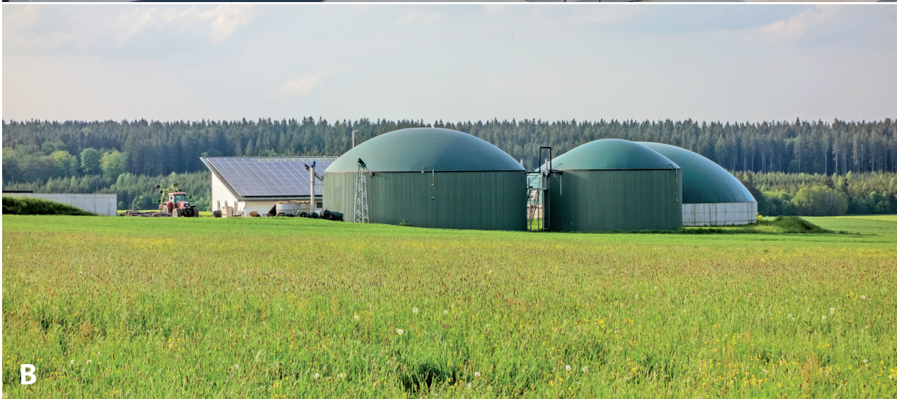
Image 12: Two examples of on-farm anaerobic digestion facilities, which provide an opportunity to recover biogas and nitrogen rich digestate (Manure Measure 11). The approach should be integrated with low emission spreading, ammonia stripping or other nutrient recovery to avoid subsequent ammonia losses. (A, Digestion for a pig farm Russia, photograph © Sergei Lukin; B, System combined with photovoltaics in Germany, photograph © Shutterstock, www.shutterstock.com, ID: 430844485).
