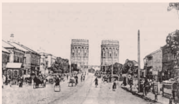
Figure 12.13 "Kretsletz" main water pumping towers.
